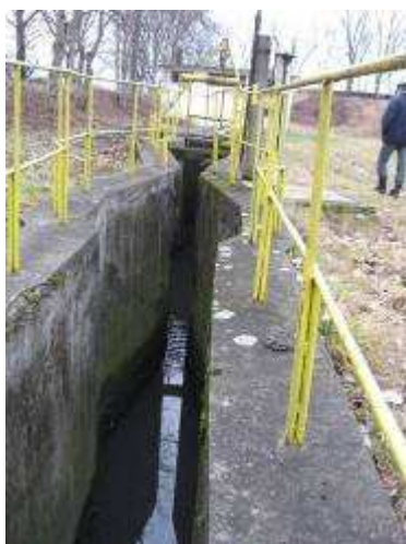
Figura 79 – Canal Parshall SEAU Reghin
