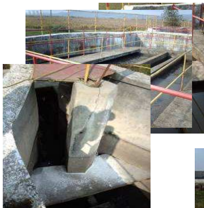
Figura 139 – Deznisipator SEAU Iernut
