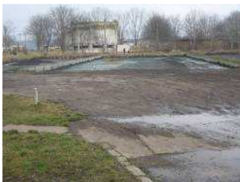
Figura 103 – Platforme uscare namol SEAU Reghin
