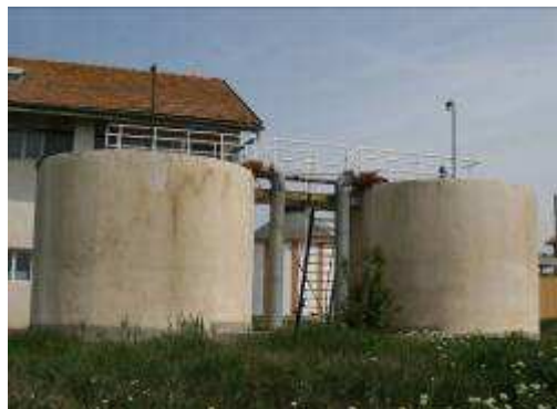
Figura 70 – Bazine tampon namol fermentat 2 x 50 mc SEAU Targu Mures
