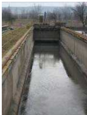
Figura 117 – Decantor primar linia veche SEAU Tarnaveni
