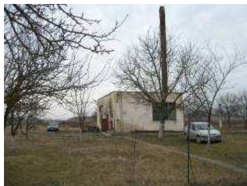
Figura 130 – Pavilion administrativ SEAU Tarnaveni
