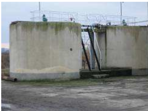
Figura 70 – Bazine tampon namol fermentat 2 x 50 mc SEAU Targu Mures
